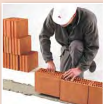
First course bedded in normal mortar
