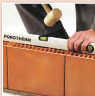
Double check levels in all directions
