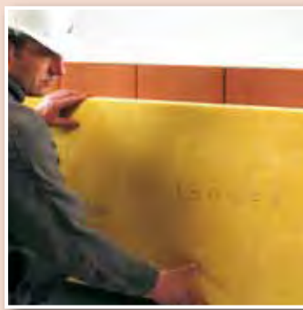
Install wall ties and fix insulation
