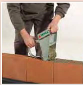
using roller tool, scoop trowel or by dipping
